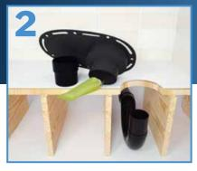
Measure and cut an ABS or PVC piece as needed to ensure a secure connection with P-trap below. Note that the drain body has an outlet of 2". (a coupling reducer of  $1\frac{1}{2}$ " is included).
