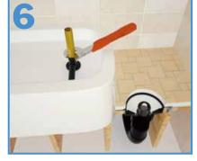
Install the piece to the tub's waste and overflow. Ensure the measurement between the base of the drain and P-trap will fit the tailpiece.
