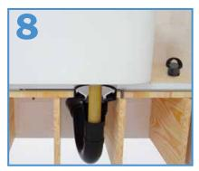
Carefully insert the bathtub tailpiece into the drain body until the bathtub is in place.
