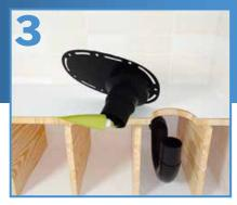
Connect the drain to the P-trap. Glue coupling reducer (if necessary) to the drain body first, then to the P-trap. Apply glue to both ends for a safe installation.
