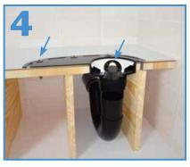
Secure the drain body to the wood floor using screws or cement. \*Temporarily insert the plug to prevent residue from entering the drain.
